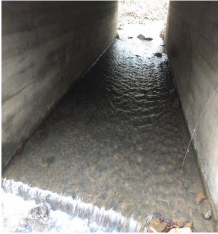
Figure 2. Fast, Shallow Water and Drop at Culvert Exit
